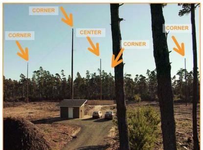
the ground to terminate the two support guys for the four corner poles as well as to terminate the four vertical elements symmetrically located around the base of the center pole. The installation crew arrived at the site at noon on the first day. The Kinstar antenna was completely installed by the close of the following day (see photograph); hence the total installation time was 1-1/2 days.
