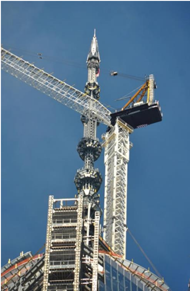
Top of spire being placed atop One World Trade Center, May 10 2013
