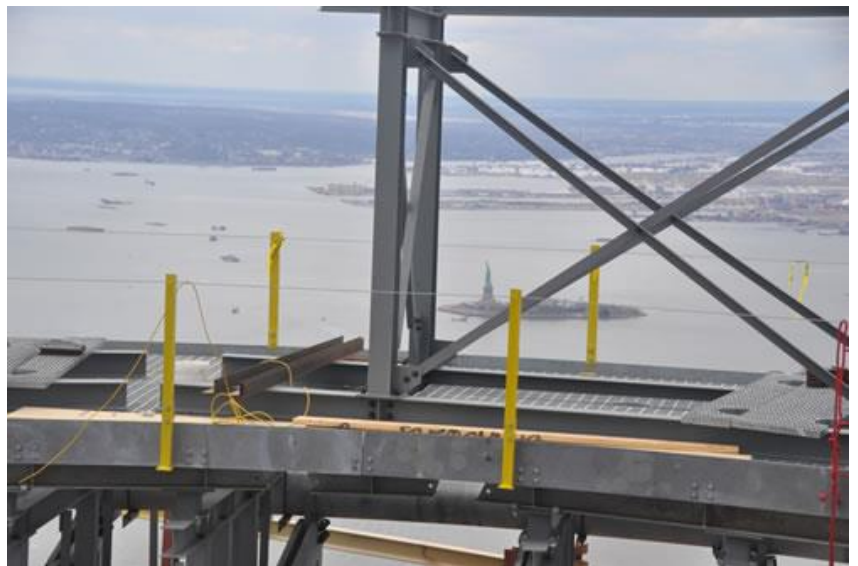
Communications Rings being installed at One World Trade Center
