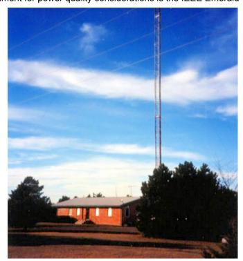
**RETROFIT OF AN OMAHA TV STATION** – KPTM-TV occupies a studio facility in downtown Omaha, Neb. Trouble started when a 365-foot tower was built adjacent to the studios to transmit the signals to their main transmitter 10 miles away (see photo below – this tower is directly adjacent to another, seen at left). Lightning events caused about \$40,000 worth of
