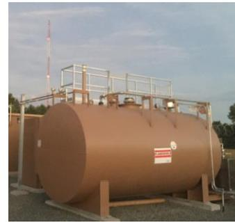
Fig 2 6,000 Gallon, Double-Walled Fuel Tank
